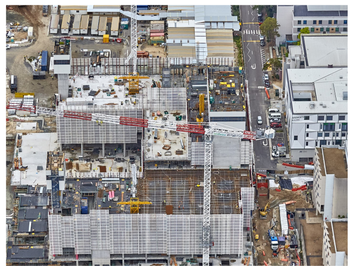
Construction activities will move to the northern end of Hospital Road towards High Street
