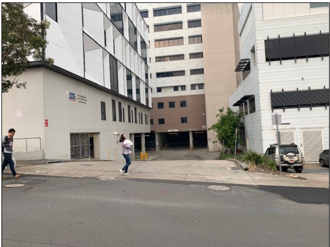
Figure 5 | View east from Hospital Road along Delivery Drive (Source: the Department)
