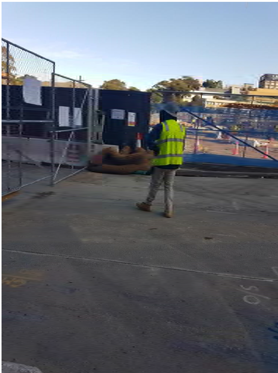
Erosion and sedimentation controls on standby at site entrance gate
