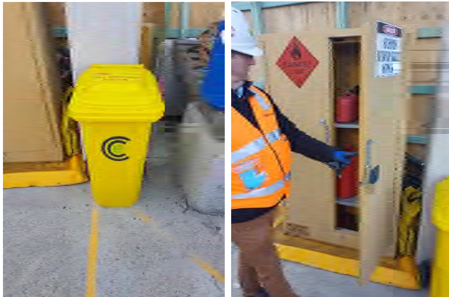
Spill kit and dangerous goods store
