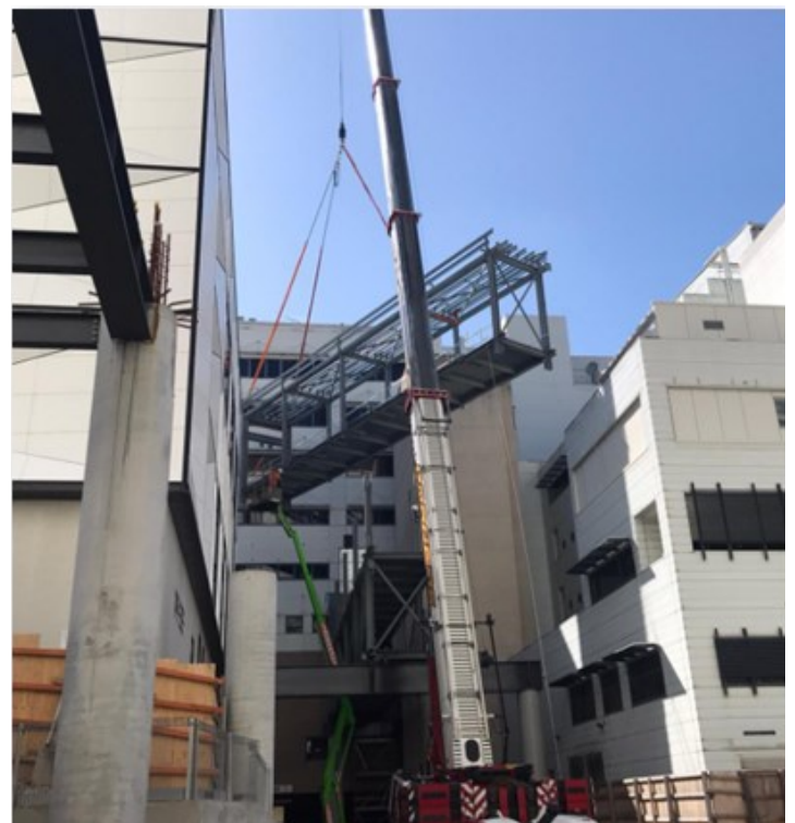
Pictured above: One of the link bridge modules arriving on site
