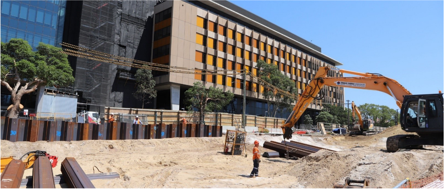
Construction workers install temporary sheet piles to allow work to commence on upgraded stormwater infrastructure along the Botany Street frontage
