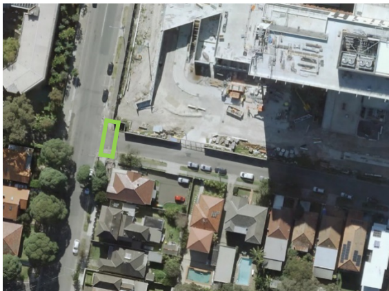
Location of potholes to be rectified on Magill Street
