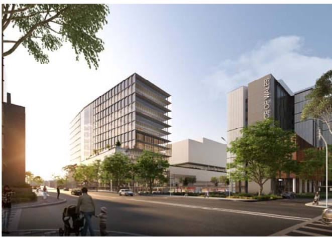
Artist's impression - Acute Services Building, Health Translation Hub and Sydney Children's Hospital Stage 1, view from Botany Street.
