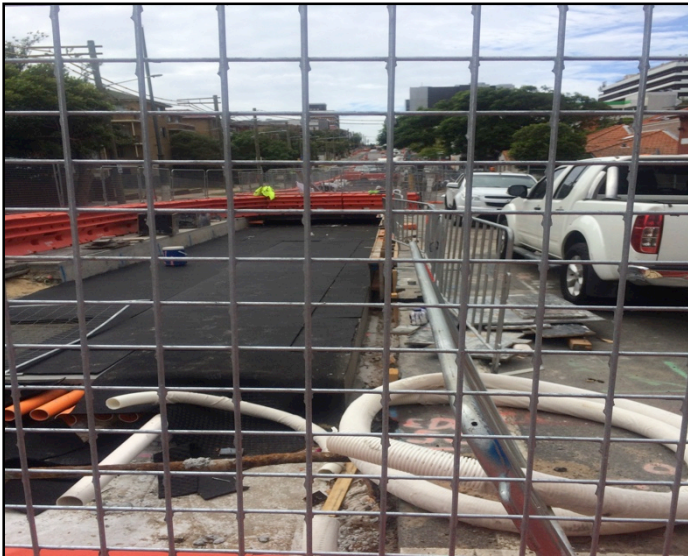
Figure 8. Light Rail construction along Street
