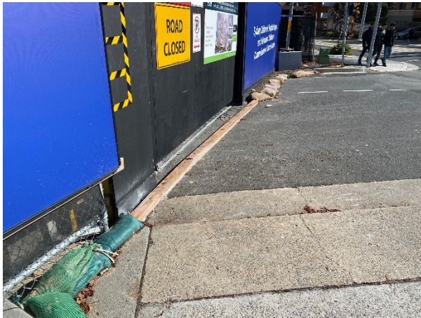
Clean water diversion adjacent to hoarding at Hospital Road. Narrow driveway into JHG site. Coir log bunding along driveway to minimise dirty water moving offsite from the driveway.
