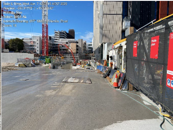
Clean water diversion adjacent to hoarding at Hospital Road. Narrow driveway into JHG site. Coir log bunding along driveway to minimise dirty water moving offsite from the driveway.
