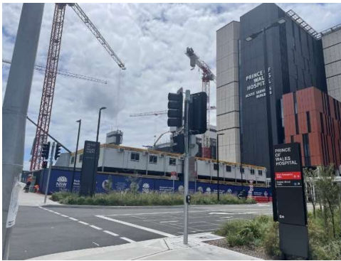
Remaining construction office and hoarding
