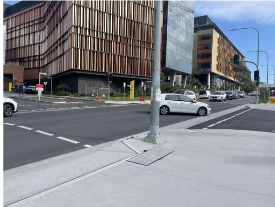
Traffic signal and wayfinding signage
