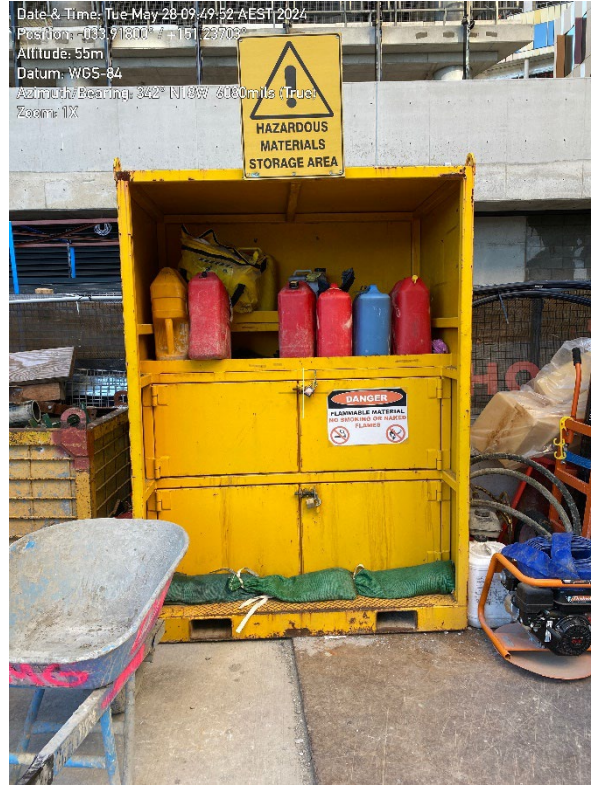
Flammable storage area.
