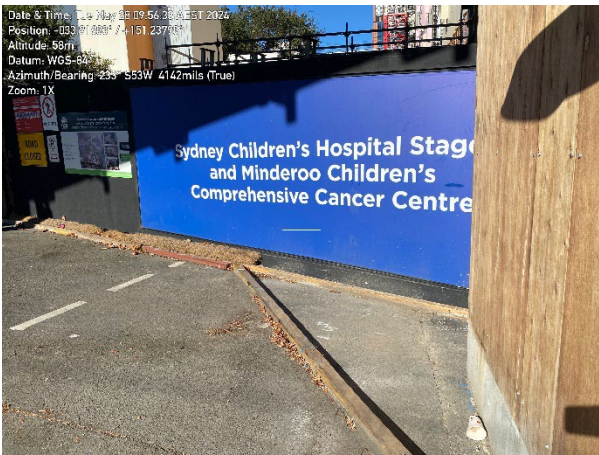
Clean water diversion adjacent to hoarding at Hospital Road.
