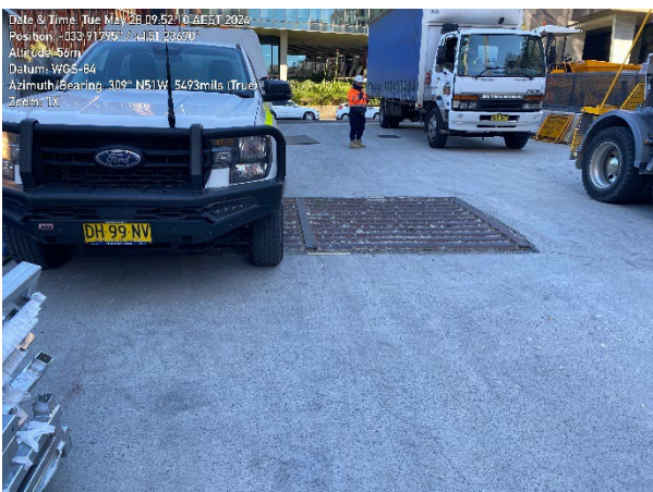
Rumble grid constructed within the temporary driveway.
