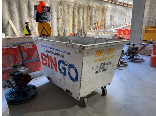
Waste bin, and clean and tidy site.
