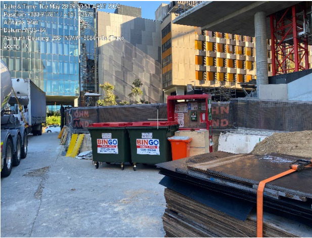
Nurse station, spill kit and waste bins along to driveway.
