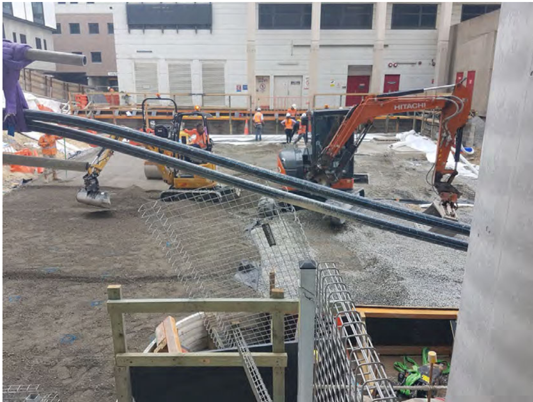
Final base layers being prepared for concrete pour
