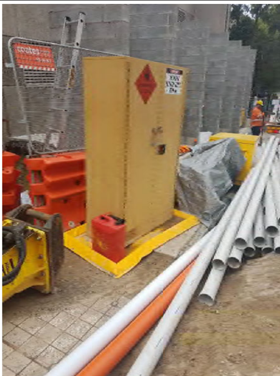
Dangerous goods store (containing fuel)
