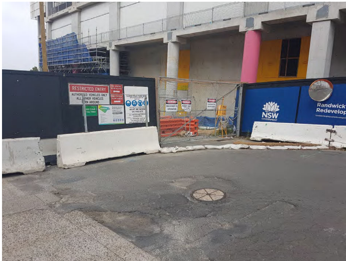
Hoarding ion place with signage
