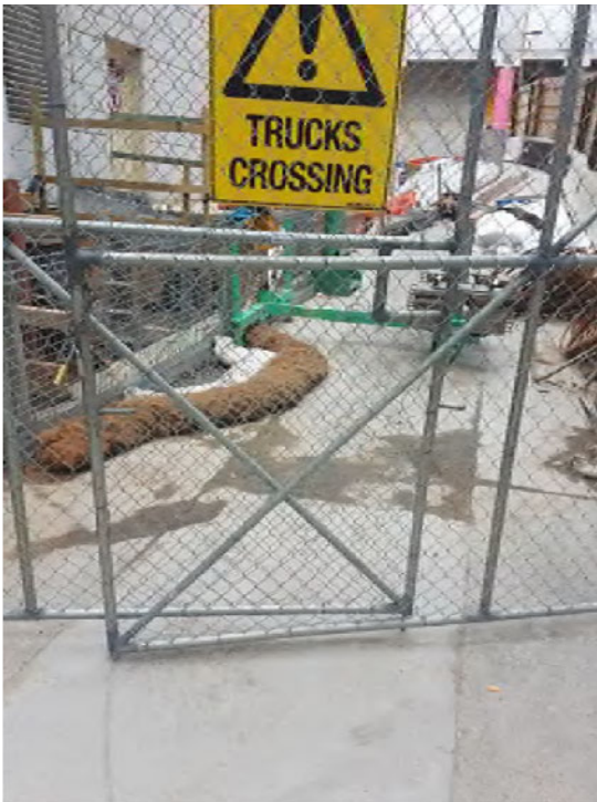
ERSED control on pit
