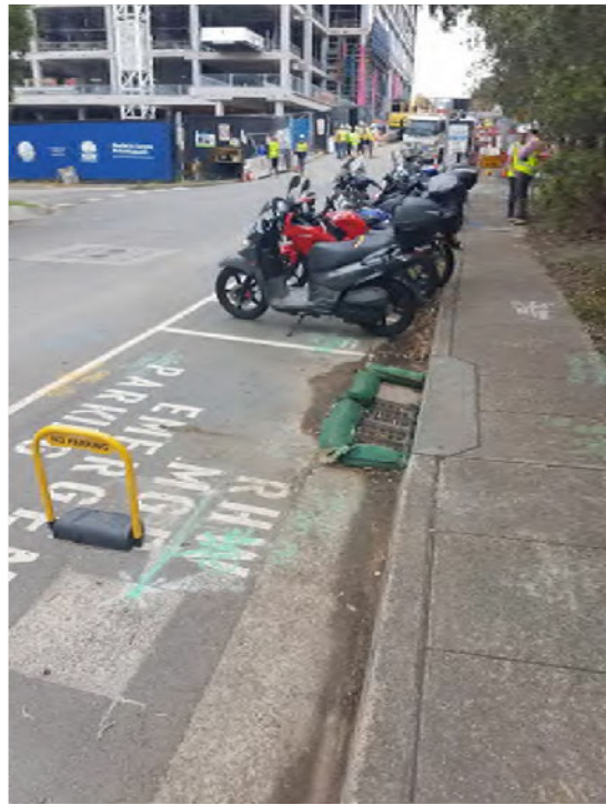
ERSED control on public road down from the site gate
