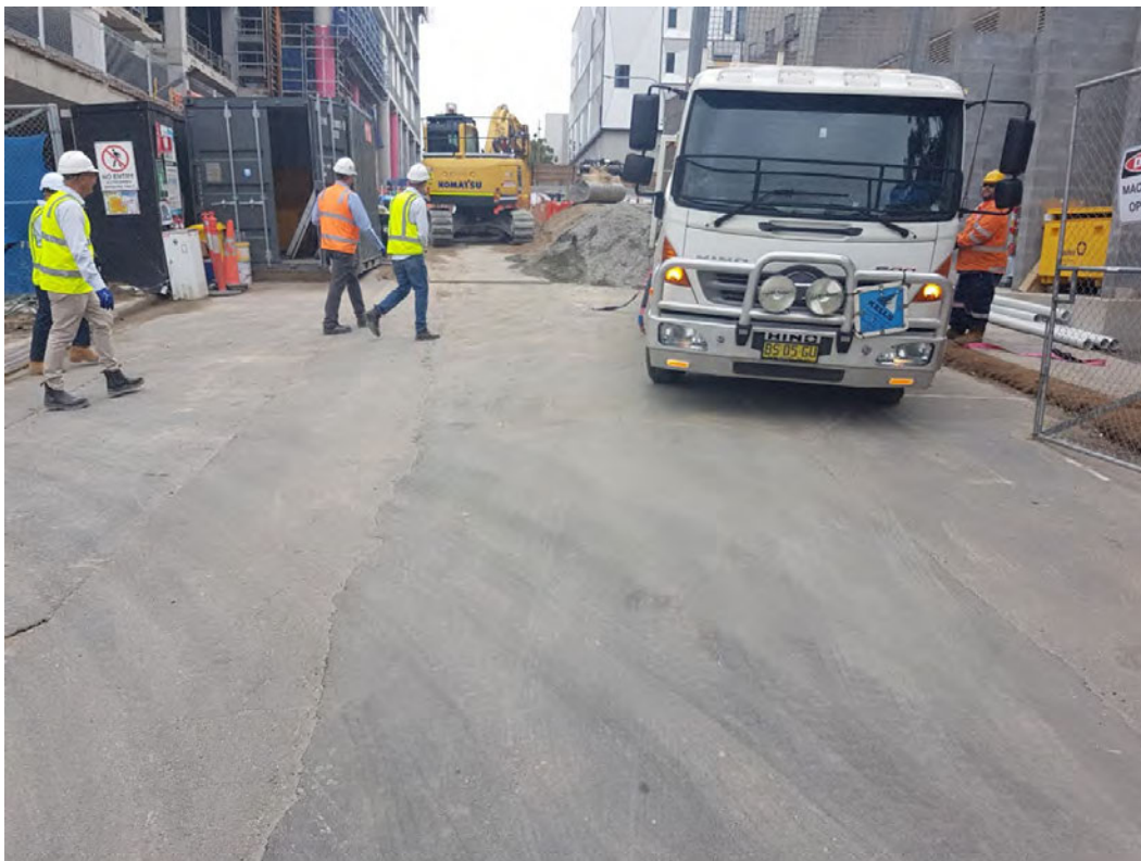
Concrete apron for vehicle parking
