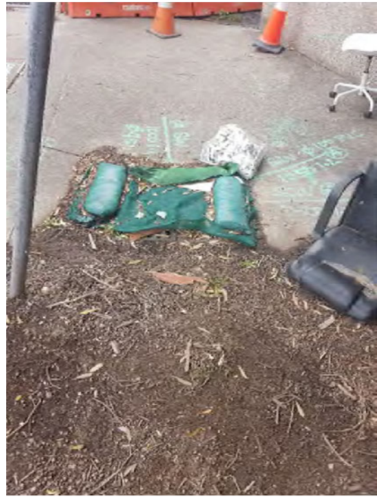
ERSED control on pit
